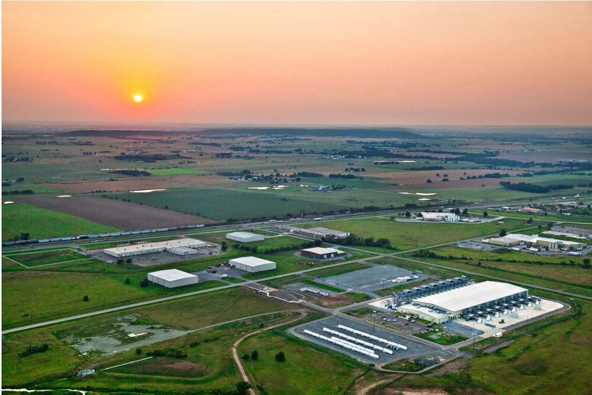
Google data centre, Pryor, OK
